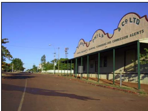
Plate 8: Burns Philp warehouse Normanton
